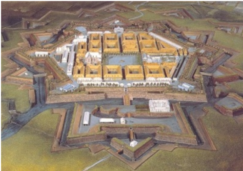
Figure 5. Vauban fortress Saarlouis with bastions at the edges
